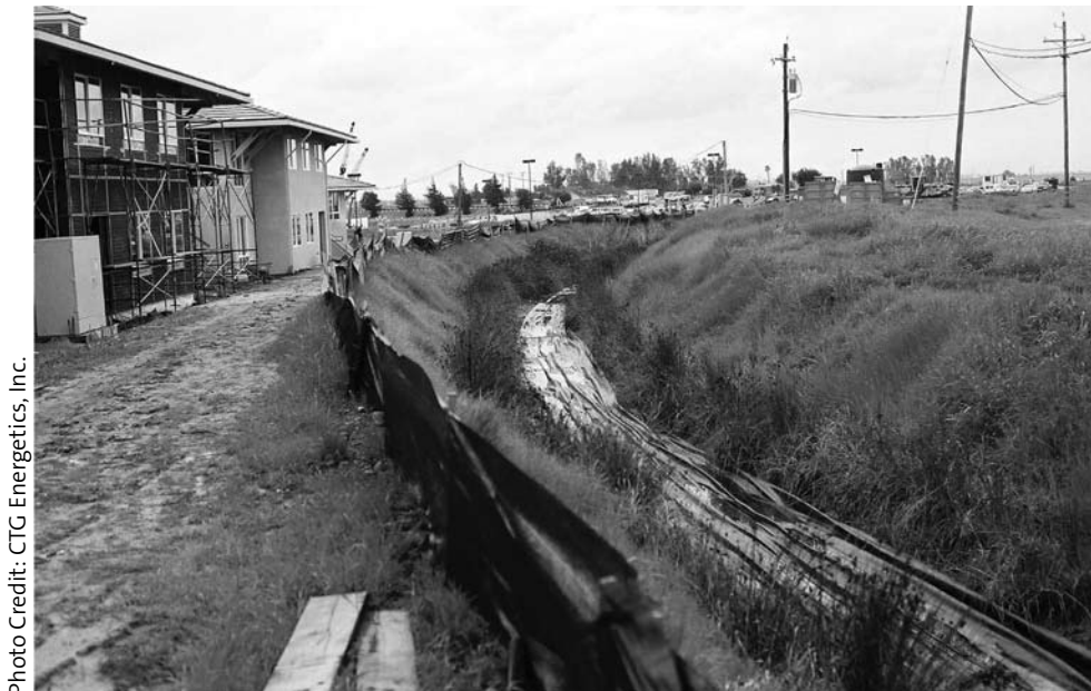
Example of Structural Control. Silt fence: fabric filter media removes sediment from stormwater volumes flowing through the fence.
